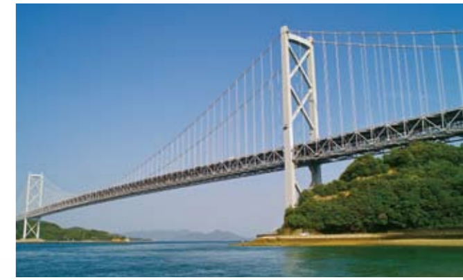
Innoshima Bridge (Onomichi City) "Innoshima Bridge" is the second bridge on the Nishiseto Expressway coming from Onomichi. The bridge has a 2-level construction and can be crossed on foot or by bicycle, making it a great place to enjoy a pleasant, hour-long walk over the sea.
